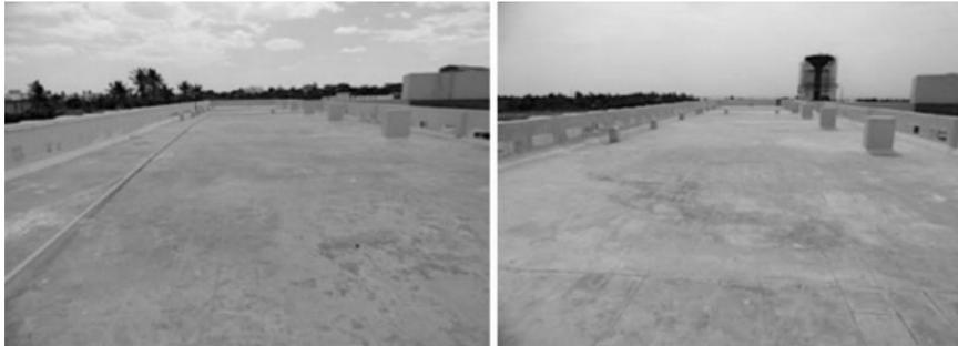
The roof area is separated 10 blocks, there are 2 types roof where one type is having water tank, thus two types design is mentioned in this project, detail design requirements is shown in Table 1 and Table 2. In accordance with shadow analysis, space has been left between two rows and sidewalls for allowing free movement of people for inspection, maintenance and cleaning.
